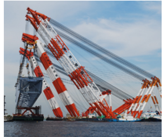
The main lift involved three floating cranes
