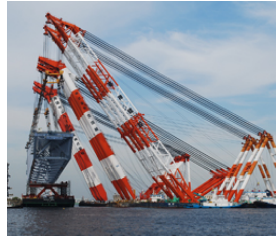
The main lift involved three floating cranes
